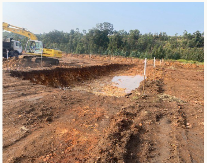
Box cutting for an attenuation pond
