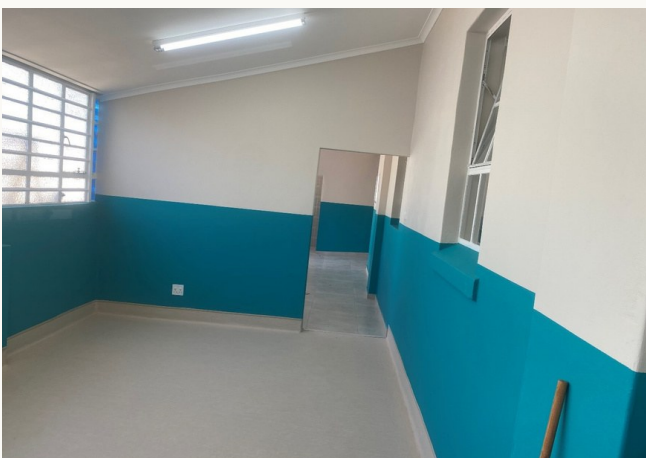
Comfort room refurbishment
