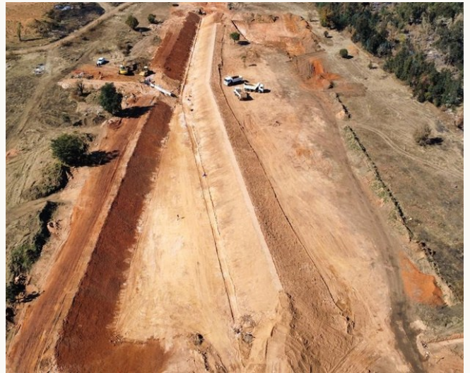
Bulk earthworks & attenuation pond
