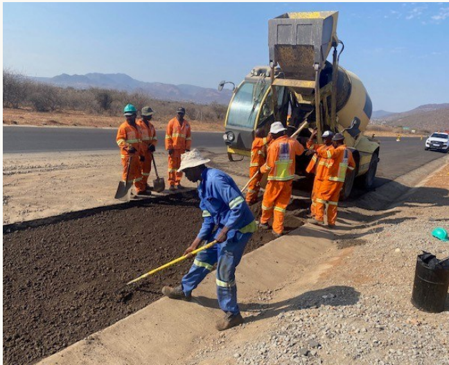
Road patching works
