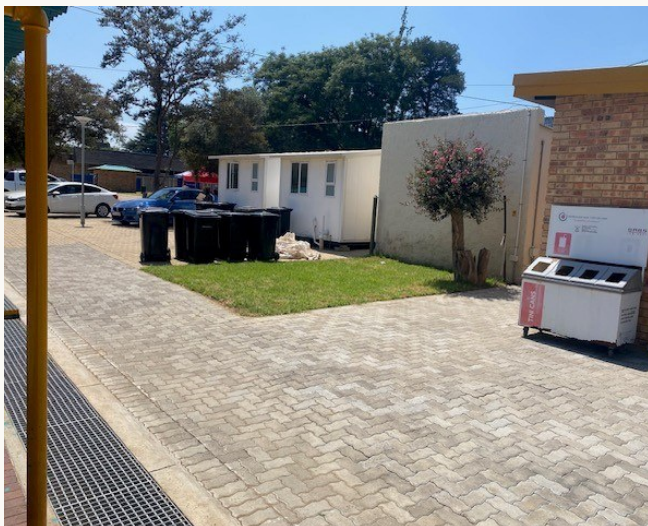
Stormwater control, paving & kerbs
