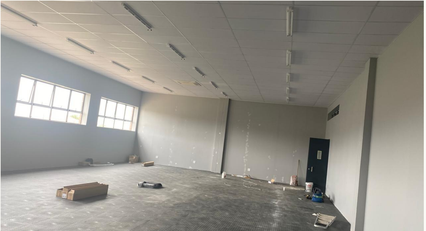
Interior refurbishment - ceilings, walls and floor preparation
