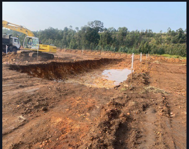
Box cutting for an attenuation pond
