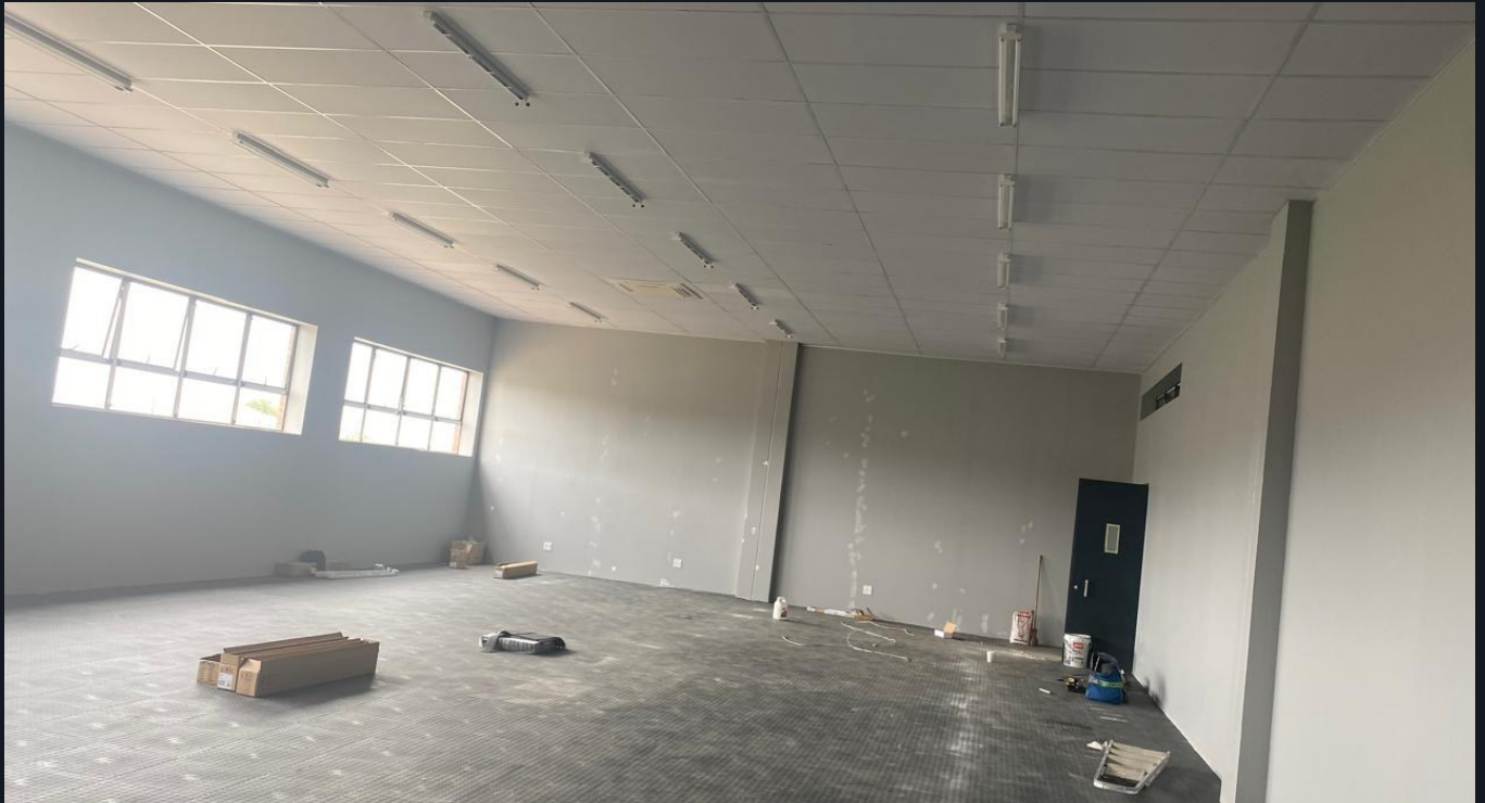
Interior refurbishment - ceilings, walls and floor preparation
