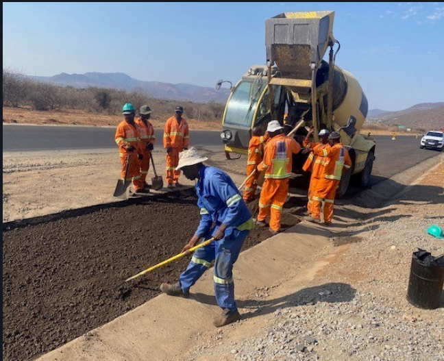
Road patching works
