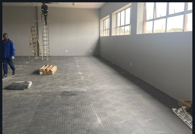
Interior works in progress
