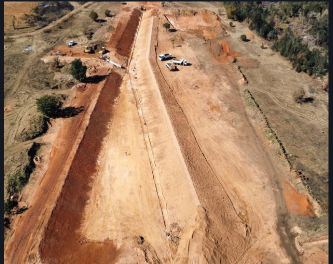
Bulk earthworks & attenuation pond
