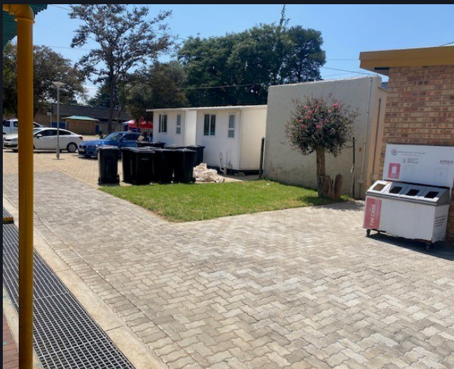
Stormwater control, paving & kerbs
