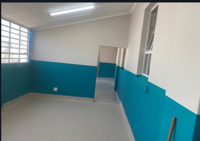
Comfort room refurbishment
